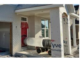
AeroBarrier was chosen as Beazer's air sealing solution for its proven ability to seal the building envelope to 1.5 ACH50 every time, verify that via a continuous blower door test, and repeat and scale that over thousands of single-family homes in different regions of the country.
